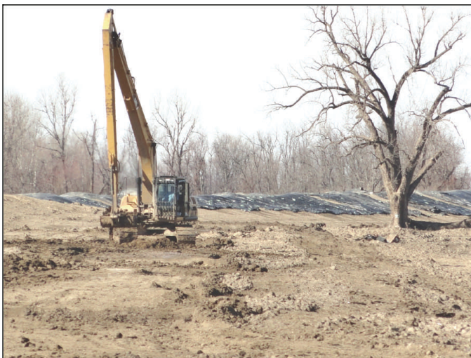
The team performs road maintenance at the center crevasse Friday. Here, an excavator removes soft spots in the road. The excavated hole will be filled with rock that will better support heavy equipment during the reconstruction of the levee.
