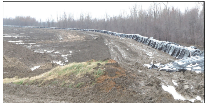
HESCO barriers span the length of the upper crevasse Dec. 15. The plastic sheeting protects against erosion and provides a water-resistant barrier.
