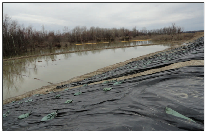
River water rises against the levee at the center crevasse Friday. With the crest passing, this segment will see 1-3 feet of water at the toe of the levee.
