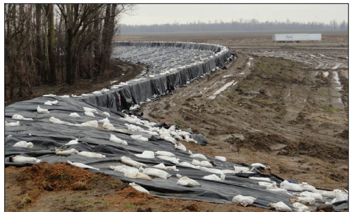
The District team completed repairs to the plastic at the upper crevasse Thursday. The team added additional sandbags to better hold the plastic in place.
